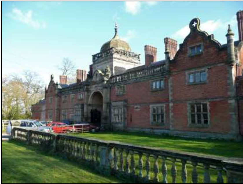
Figure 18. Ingestre New Stables showing central entrance tower
