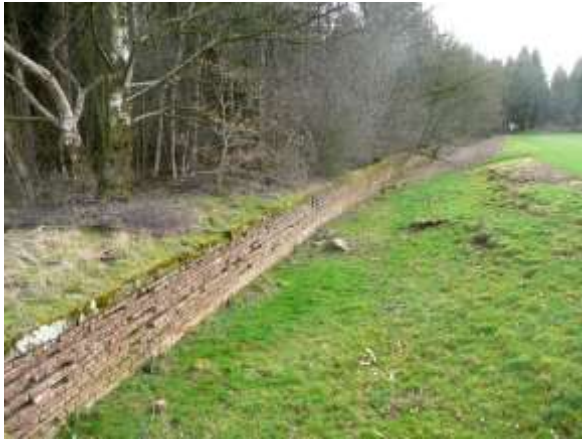
Figure 46. Brick Haha at the edge of Ingestre Wood
