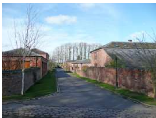
59. Entrance to Home Farm Court development showing street light on right
