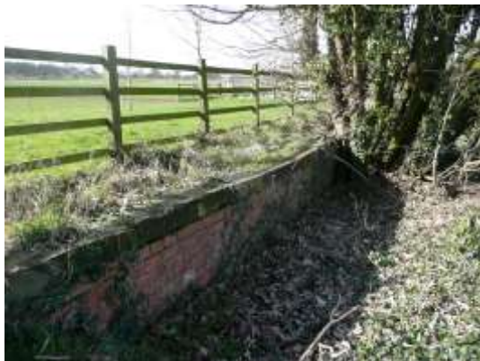
Figure 48. Stone topped wall along track leading from Home Farm to Trent Drive
